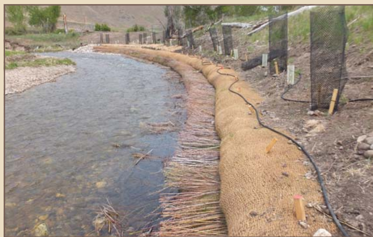
Before and after photos of second project site: bioengineered bank with live brush toe and native vegetation plantings
