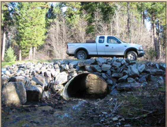
Culvert installed on lower Fawn Creek, (tributary to the Fisher River) to improve fish passage and reduce risk of culvert failure.
