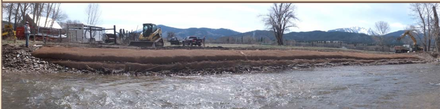
Before and after photos of first project site: encapsulated soil lift, live brush toe, and native vegetation plantings
